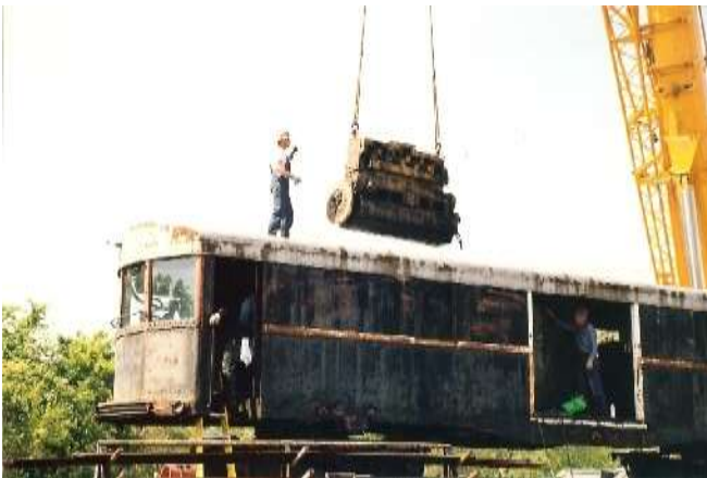
TSRR crews unloaded and dismantled Car 646.
