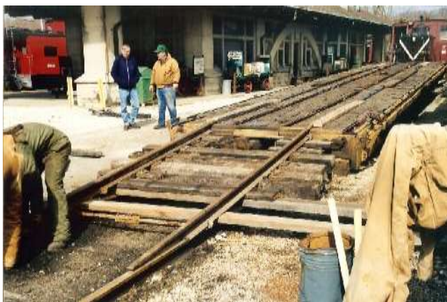
Special track work created a ramp.
