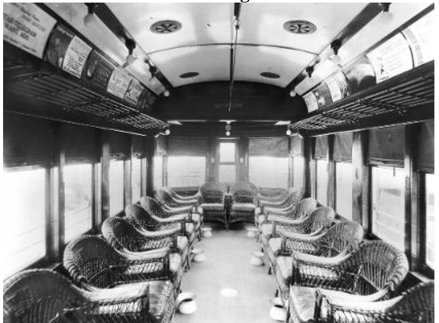
Rear compartment of car 411 showing newly installed wicker chairs, gloss white ceiling, and frosted globe style light bulbs.
